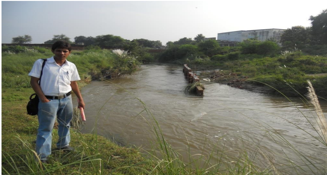
Photograph -1 shoes the construction of wall in the valley of Basna drain
