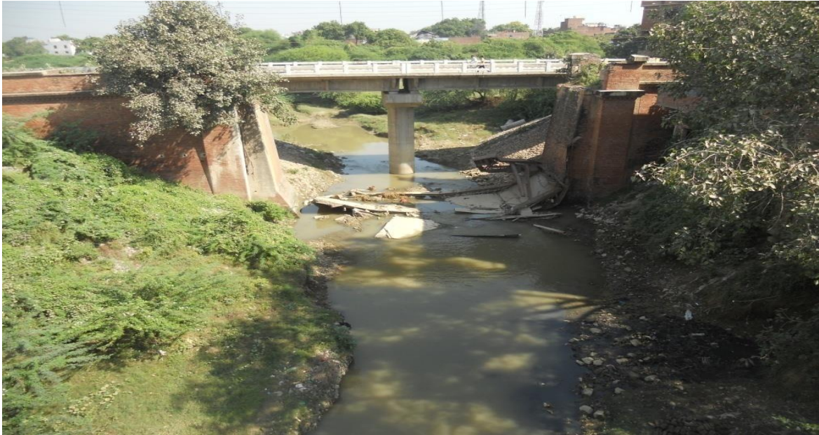
Photograph –3 shoes the collapse bridge in Basna drain.
