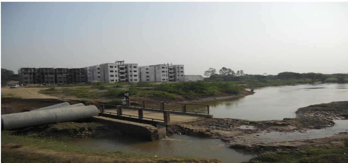
Photograph -2 shoes the incomplete bridge on Basna drain.
